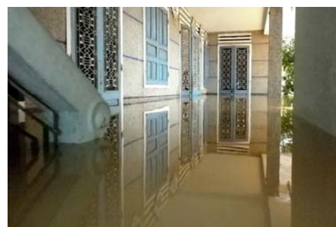
The flood rose to half of the door
